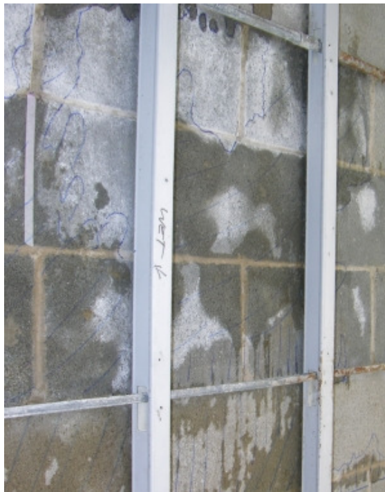
Interior view of the results of the masonry water spray test
